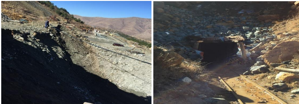
Figure 1. Erozion, soil degradation and contamination by the sterile waste of chromite mines (Photos by E. Laçi)
