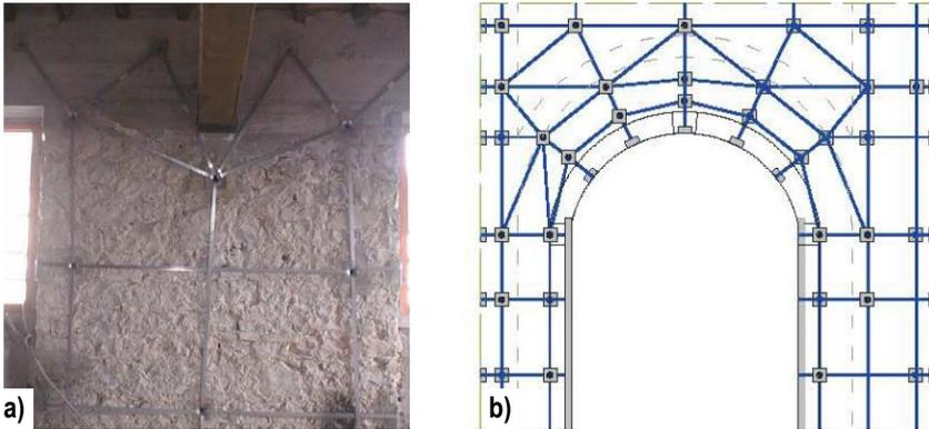
Figure 30. The use of unstructured triangular grids for a) Overcoming a truss-beam; b) Adapting the CAM net to the profile of an arched-shaped opening (Marnetto et al., 2014).
