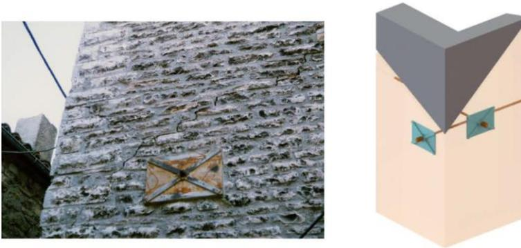
Figure 23. Umbria-Marche earthquake in 1997 (Italy): sliding-plane just over corner tie rods (left); scheme of corner detachment (right) (Marnetto et al., 2014).
