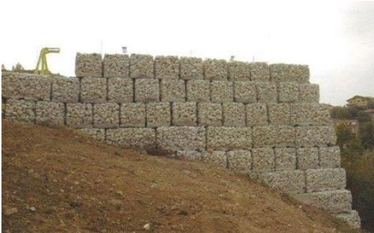
Figure 26. Metallic gabions for retaining walls and slope stabilization.
