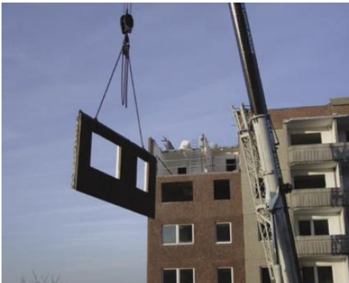
Photo 5: Dismantling of prefabricated houses.
