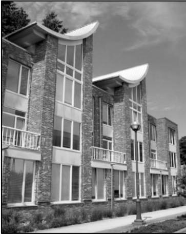
Figure 3.16. Externally reclaimed bricks, C.K Choi Building
