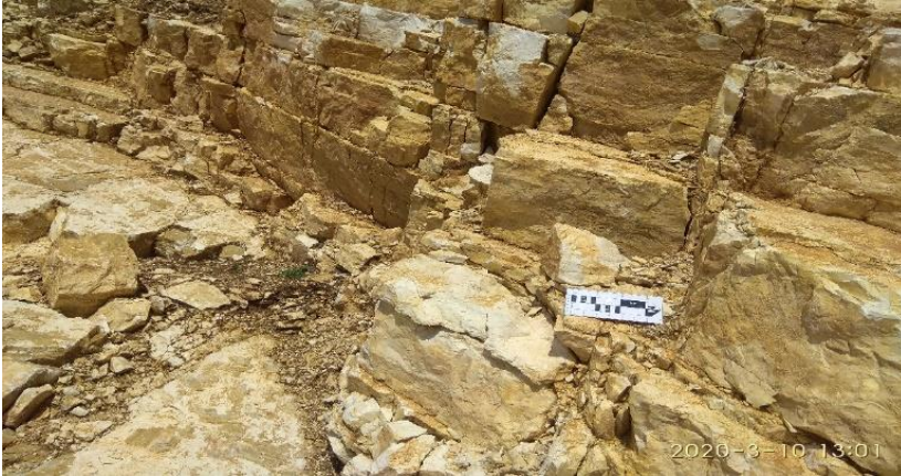
Figure 9. Orientation of the main joint sets.
