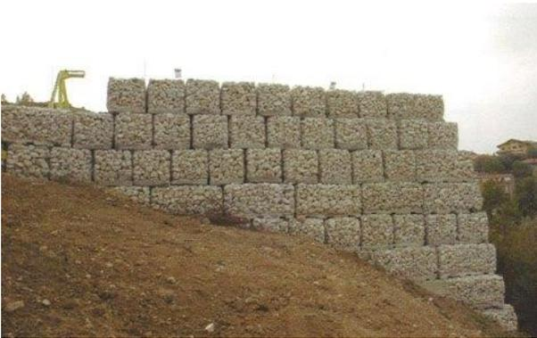
*Figure 18.* Metallic gabions for retaining walls and slope stabilization.
