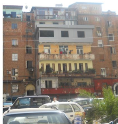
Figure 2. Building constructed before '90. Facade
