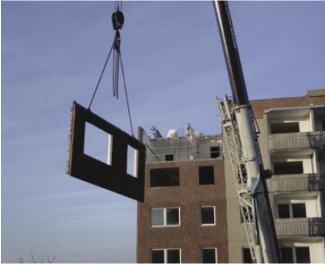
Photo 5: Dismantling of prefabricated houses.
