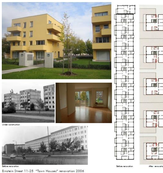
Photo 8: Successful reconstruction of apartments.
