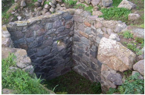
Picture: 8. Repaired bathroom. Smyrna.
