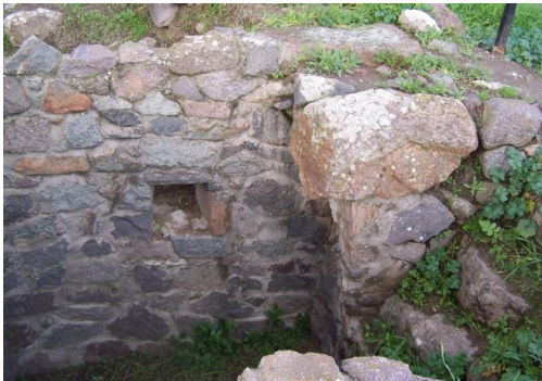
Picture: 9. Repaired bathroom space. Smyrna.
